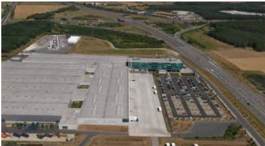
Fig. 7.28 New distribution center in Ludwigsfelde (© OTLG GmbH & Co. KG)
